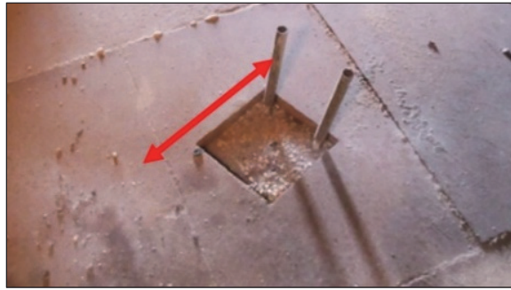
Figure 3. Slide gates with attached bar. Workers open and close sump gates to move rod and break up grain.
