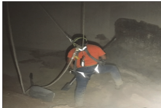
Figure 7. Example of worker breaking up towers from inside bin.
